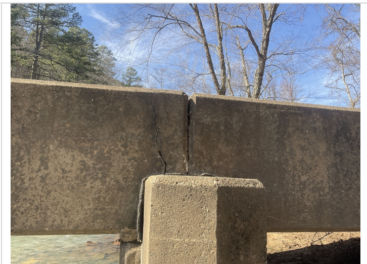
Bent 4 has vertical and diagonal cracks in the edge of slab on the right side, left side is typical.
