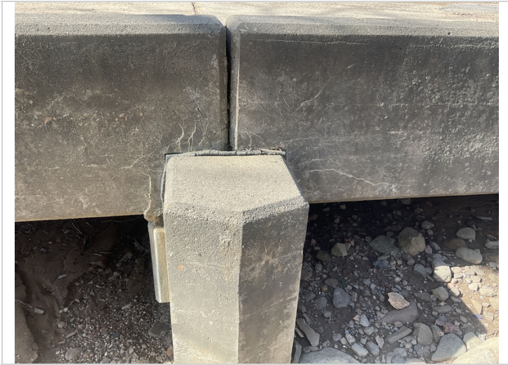
Bent 5 has diagonal cracks in the edge of slab on the right side, the left side is typical.
