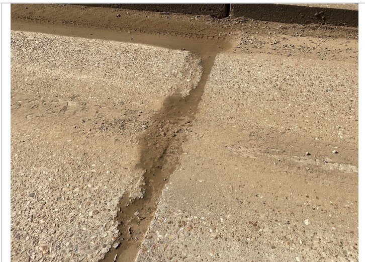
Joints are impacted with dirt.
