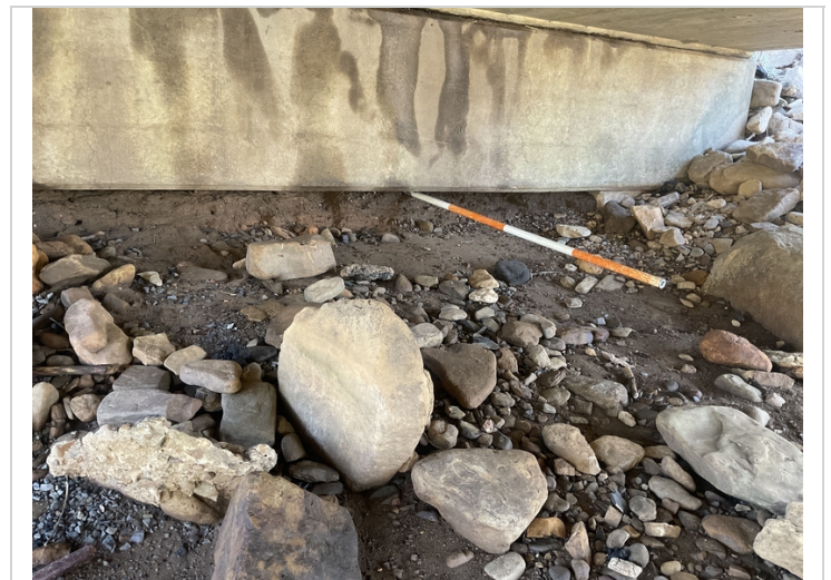
Abutment 1 has approximately 1ft of undermining under abutment cap, this is approximately 8ft in length, also there is 1 exposed concrete pile.
