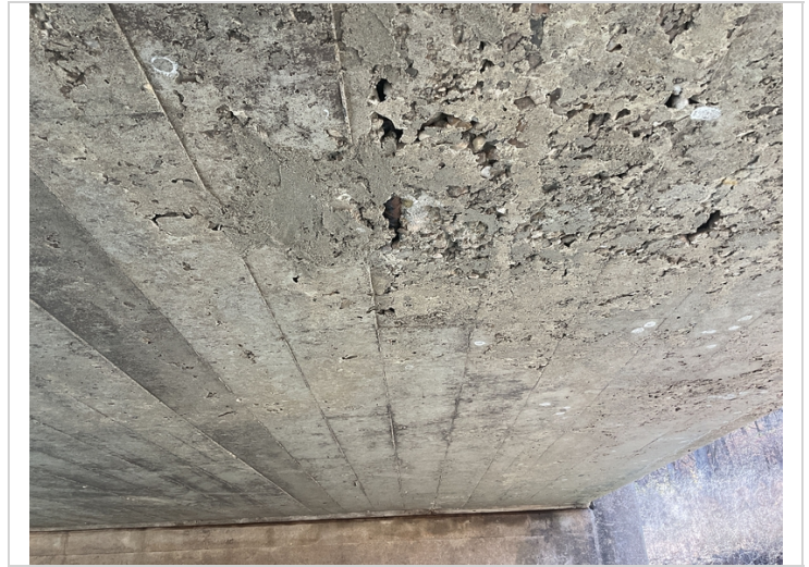
Span 3 soffit has 1 area of exposed reinforcing steel.
