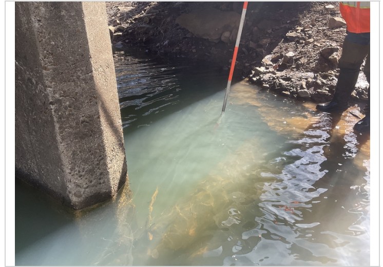
Spans 1 and 2 is approximately 4ft deep around bent 2 but there is no undermining.
