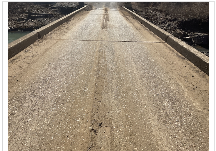
Minor abrasion throughout deck, there is exposed aggregate throughout the deck but it is still attached.
