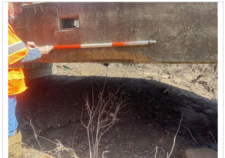
Span 4 has a large spall with exposed reinforcing steel, reinforcing steel has no section loss.
