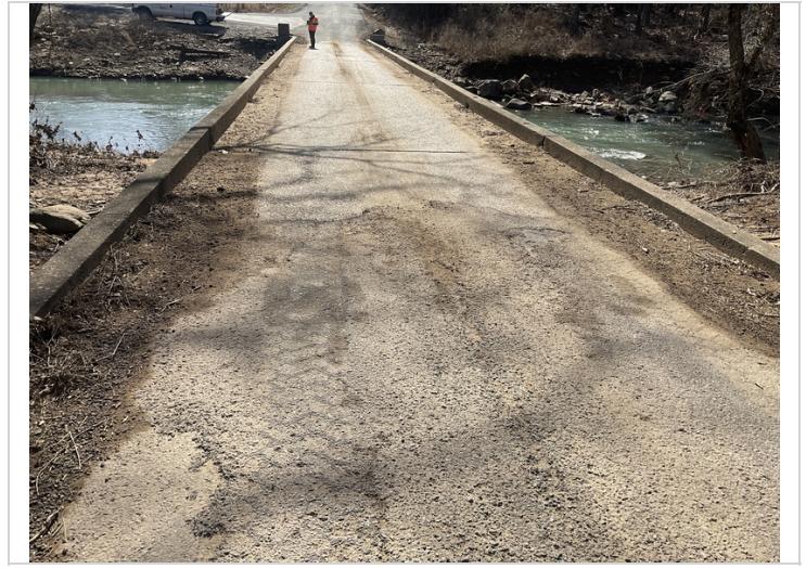
Spans 1 and 5 has asphalt that lays approximately 10ft onto the deck.
