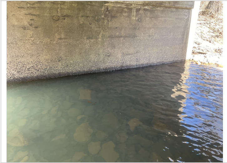
Pier walls have minor abrasion along the flow lines.
