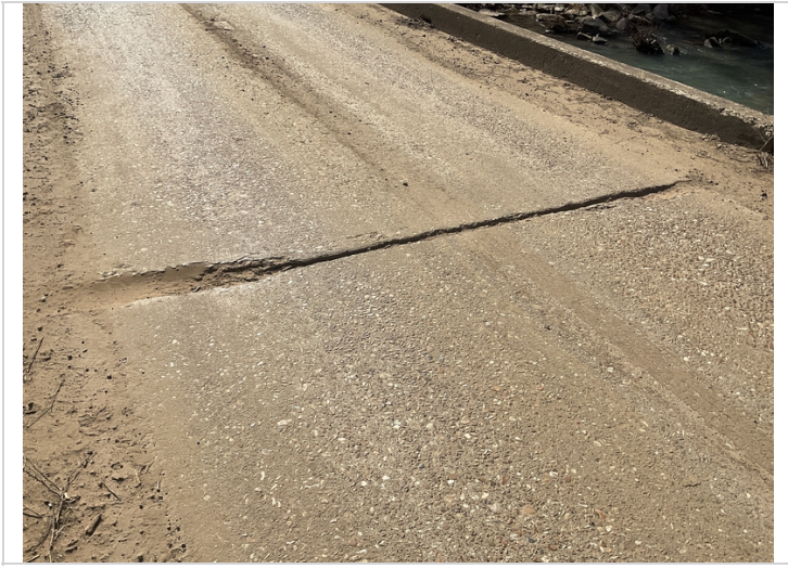
Bent 4 has 2 minor spalls along the edge of the joint.
