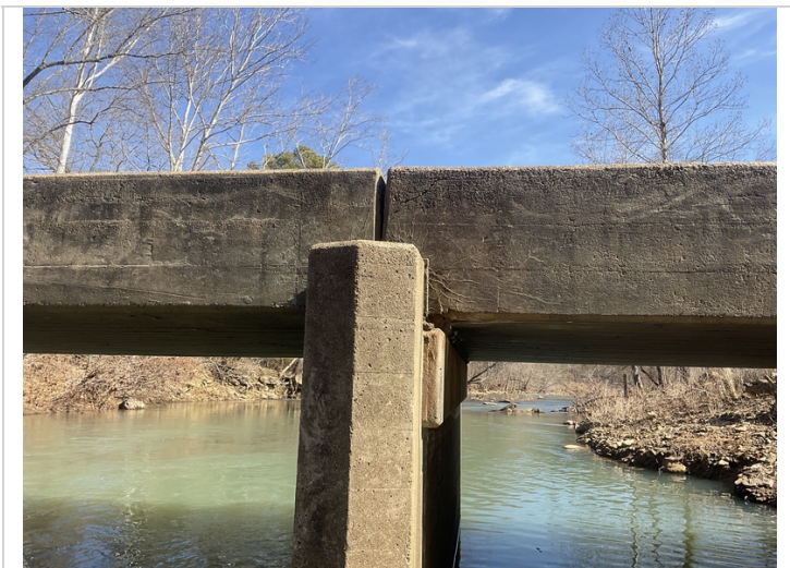
Bent 2 has vertical and diagonal cracks in the edge of slab on the left side, this is typical at all bents.
